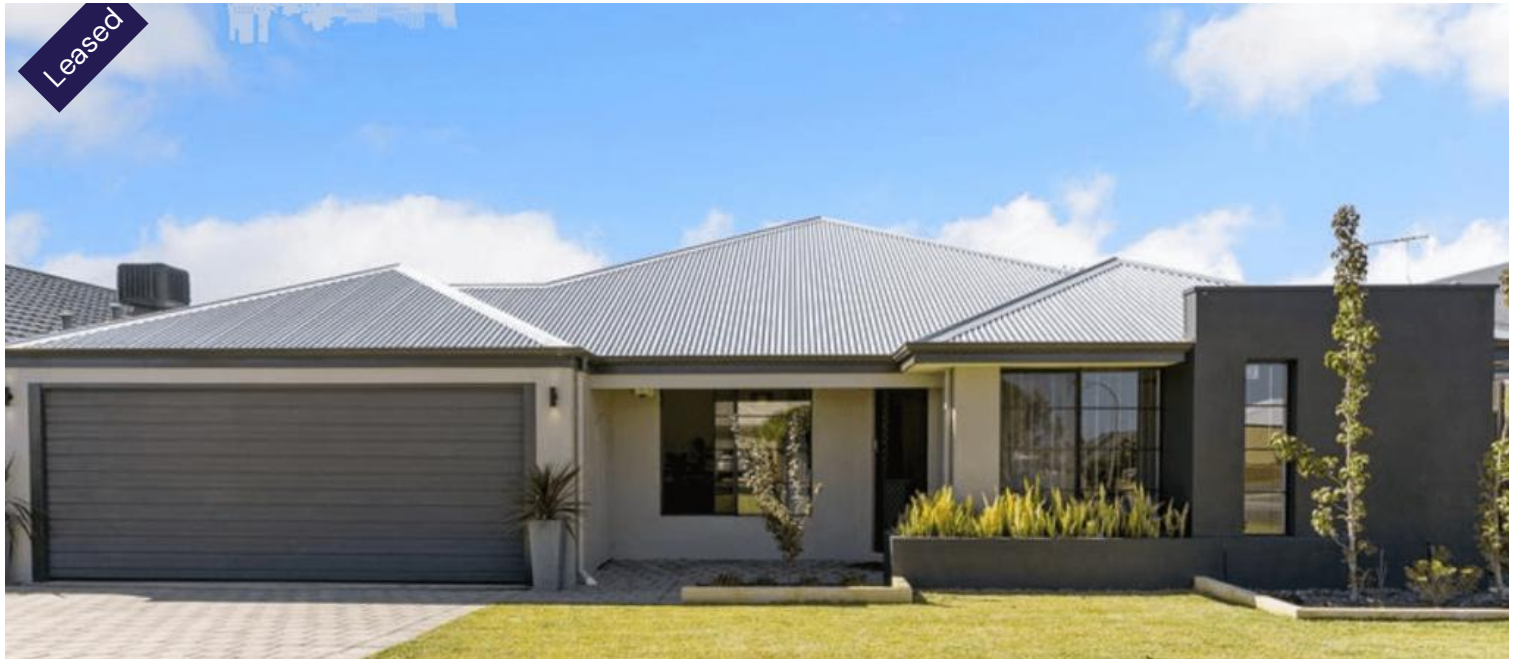
5 Inlet Link, Baldivis
